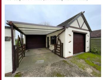
An initial open fronted car port with timber field gates and pitched polycarbonate roof.
